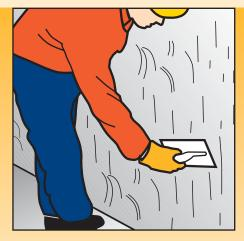
The 2nd and 3rd wall coats of Sika®-1 Render and Finishing Mortar are trowel applied to a minimum 6mm per coat.
