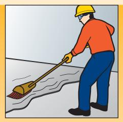
13. A Sika®-1 Bonding Coat Mortar is brush applied as a slurry to the prepared floors.
