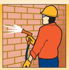
Immediately prior to installation of Sika®-1 Waterproofing System, saturate the surface with clean water.
